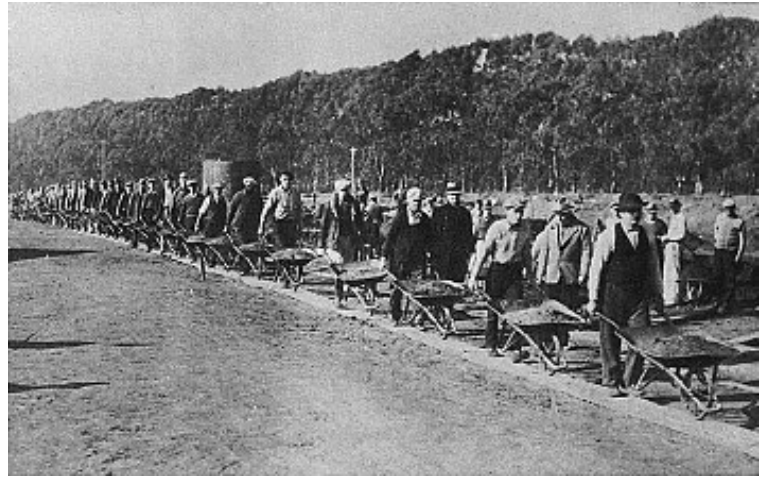
Men building a new road
